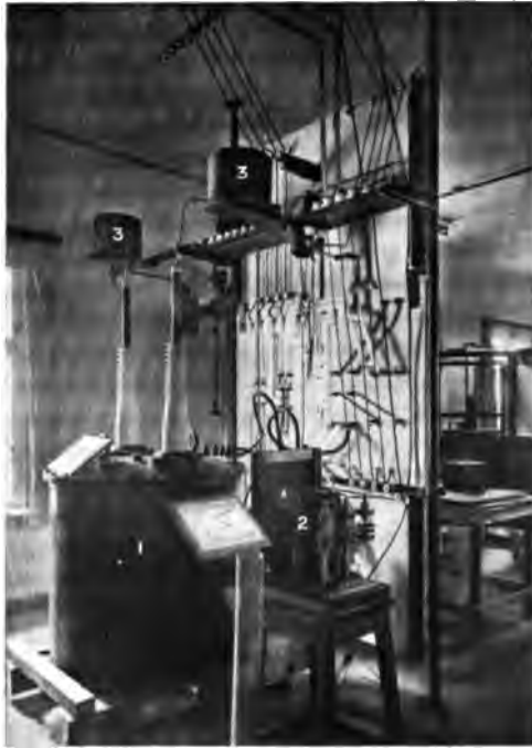
FIG. 146.—Back of switchboard of 35 T.K. station.
